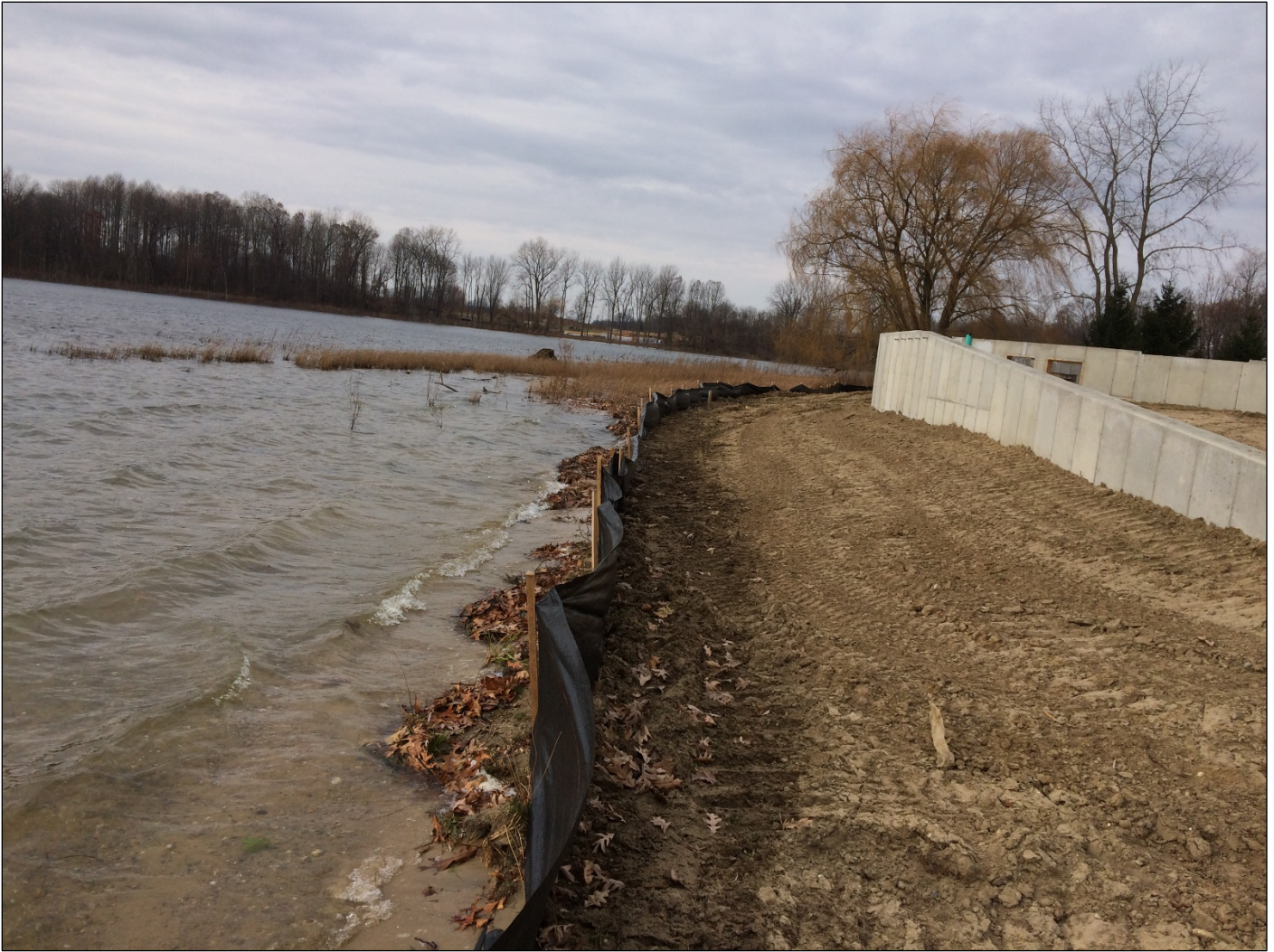
December 4, 2017 (SESC Permit Inspection) Miracle Camp
