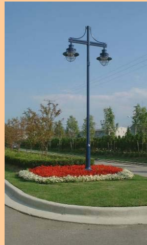
Kalamazoo Corridor Streetscape and Safety Enhancements
