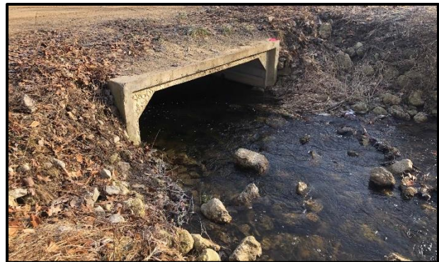
Existing Box Culvert – Looking Northeast
