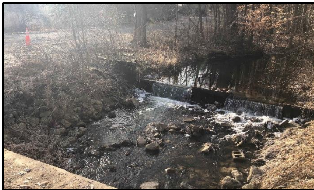
Existing Dam Structure – Looking Southeast
