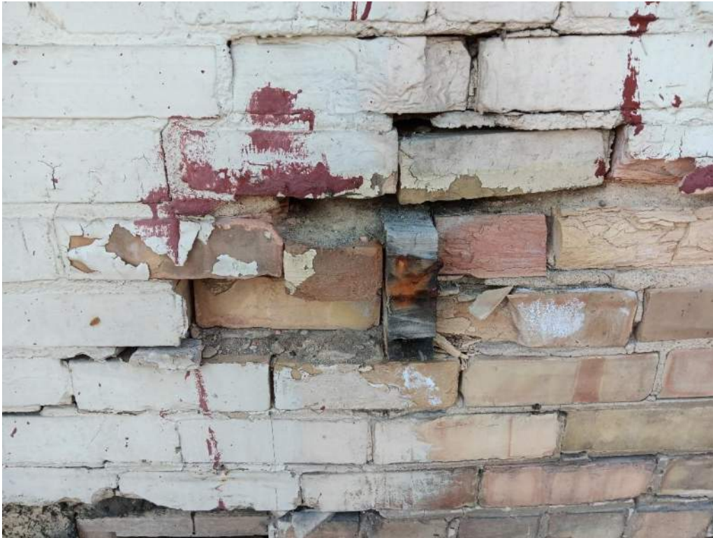
Photo 7: Floor framing embedded in brick wall.
