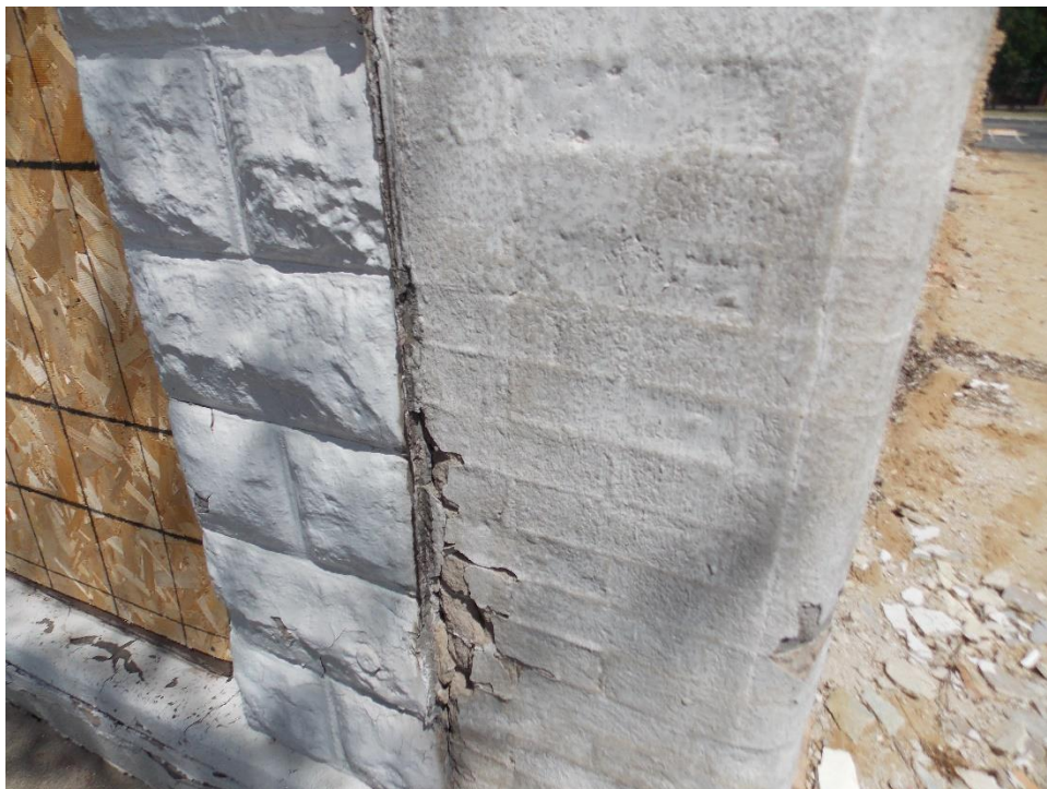
HA-06: Building Joint Caulk
