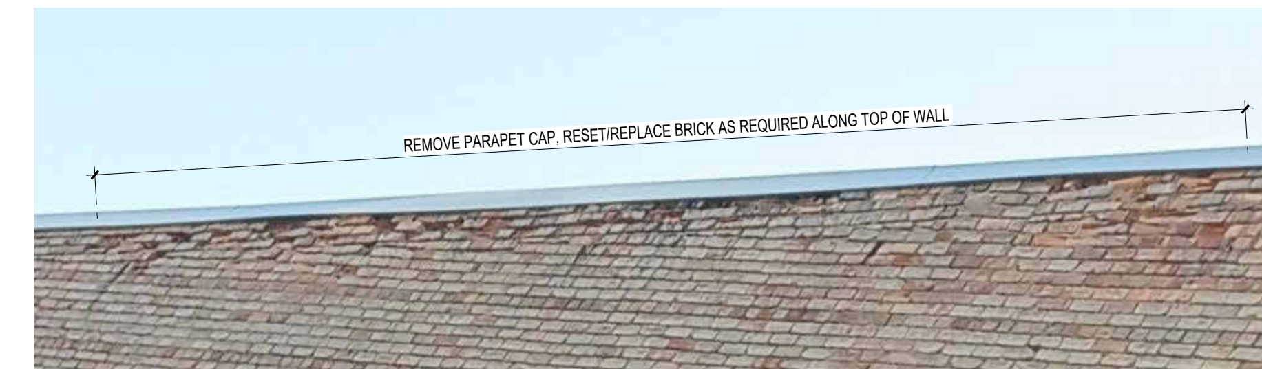
4 REPAIR DETAIL S2 SCALE: 1" = 1'-0"
