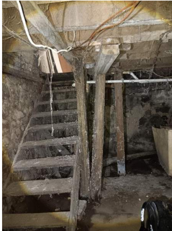
Photo 1: Floor framing at lower level stair.
