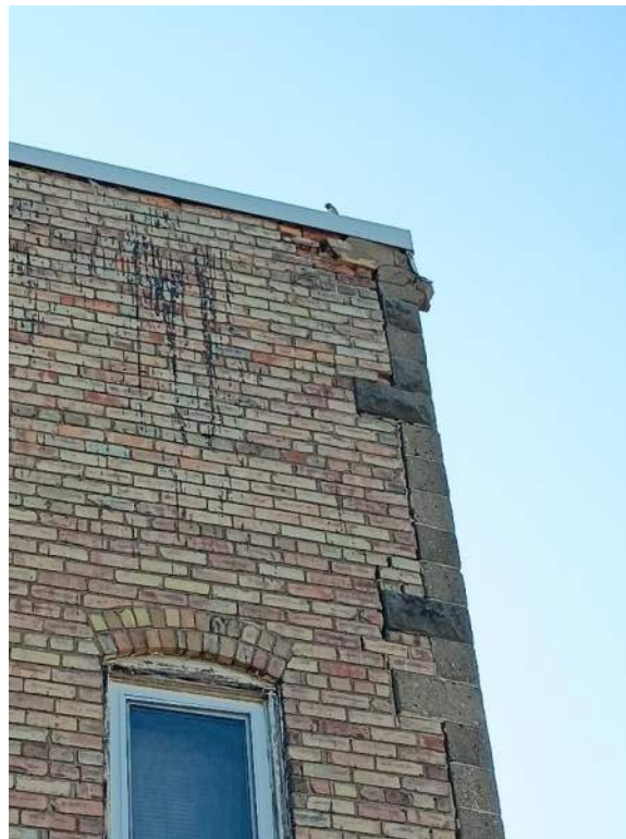
Photo 8: Southwest corner of the building. CMU wall appears to be separating from the brick wall.
