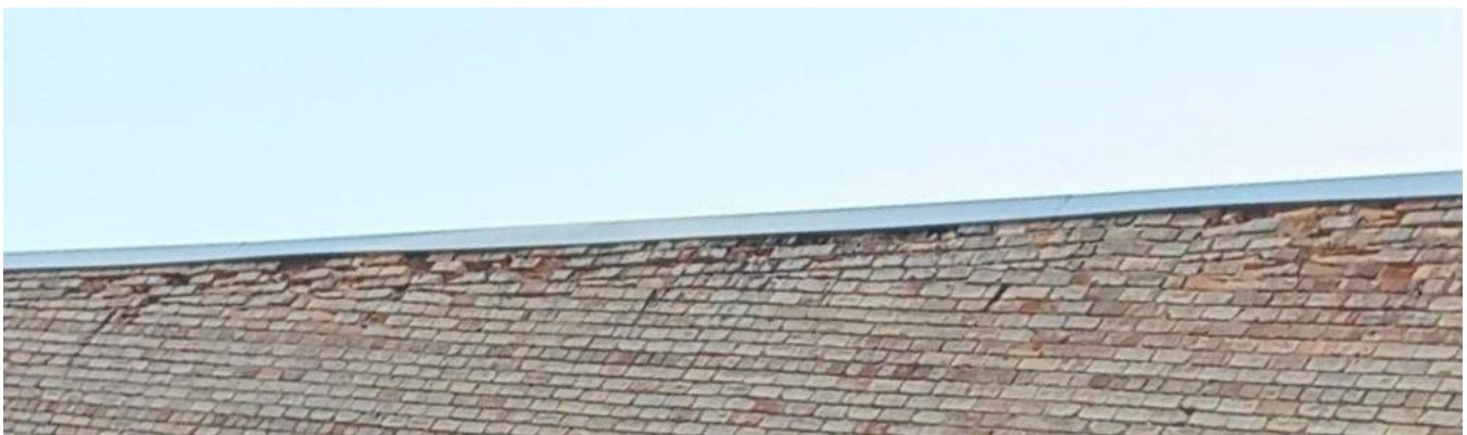
Photo 2: Top of parapet along west side of building.
