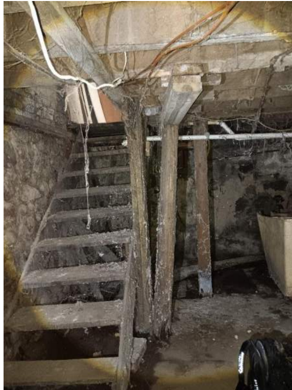
Photo 1: Floor framing at lower level stair.
