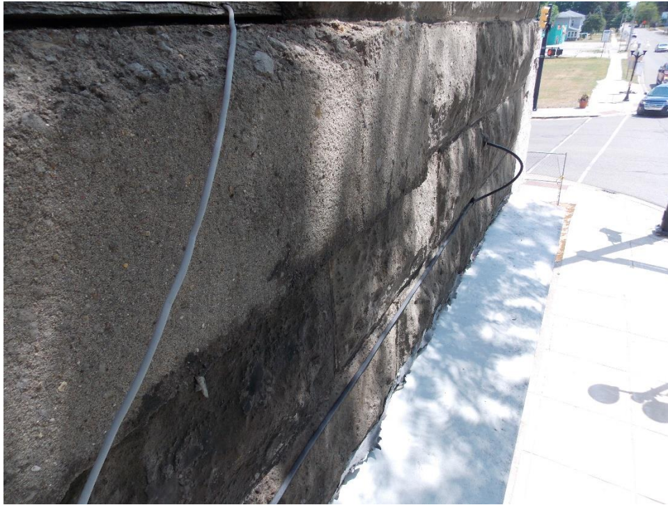
HA-04: 2nd Floor Flashing Tar
