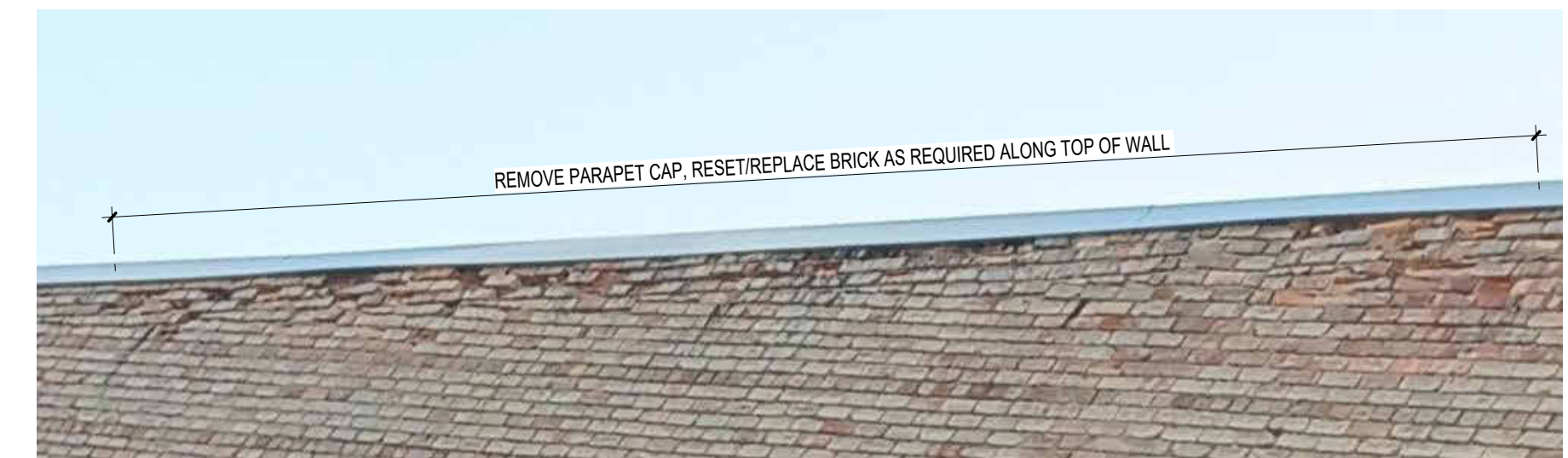
4 REPAIR DETAIL S2 SCALE: 1" = 1'-0"
